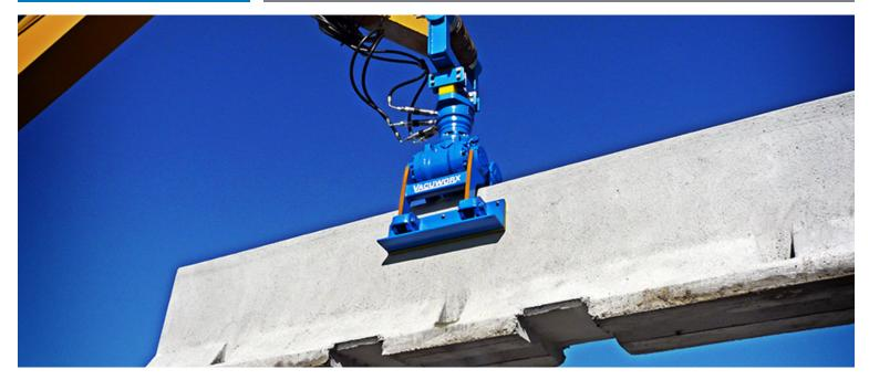
**HL SERIES HYDRAULIC LIFTERS** are designed to improve safety, boost productivity and reduce operating expenses when moving and installing concrete road barriers up to 30 ft (9 m) long and 23,200 lb (10.5 tonne). With 360° rotation capabilities, Vacuworx hydraulic barrier lifters are perfect for maneuvering in confined spaces during road, bridge and highway applications. The lifters operate using the hydraulic system of the host machine.
